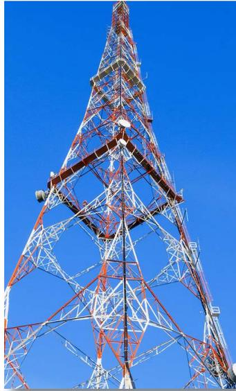
the tower almost horizontally so that as much area as possible is covered. This minimises the signal strength at ground level near the tower. The higher level RF EME therefore occurs at a height not accessible to the general public.
