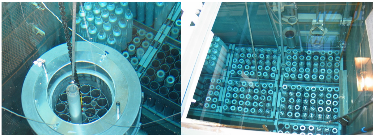
Figure 5: Wet storage facilities used for former HIFAR reactor spent fuel
