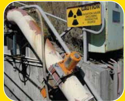
Industrial gauges containing radioactive sources installed on pipes for process measurements
