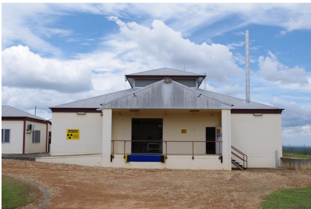
Figure 5: Queensland Radioactive Waste Store
