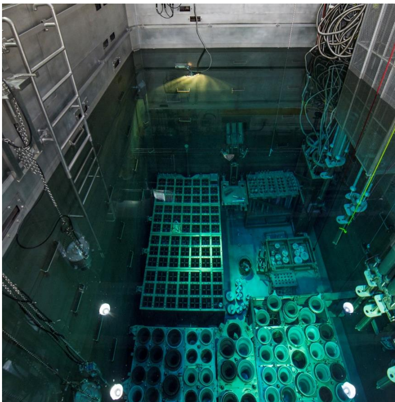
Figure 6: OPAL Reactor Service Pool including spent fuel rack storage
