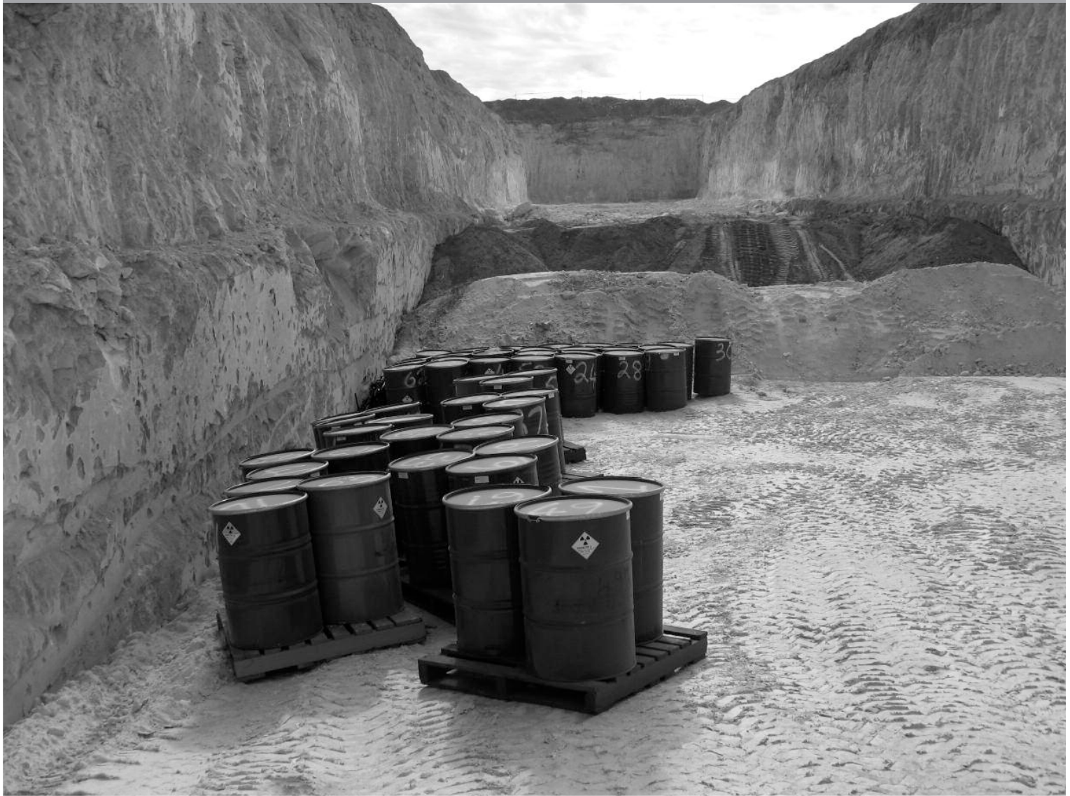
Preparing for the disposal of concreted and drummed radioactive waste in a near-surface disposal facility. Image credit: Stuart Woollett
