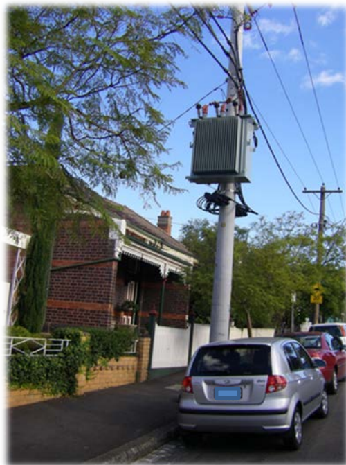
Pole mounted transformer located at approx. 25 Gower St Kensington. There are residential properties on all sides of the transformer and a primary school nearby.
